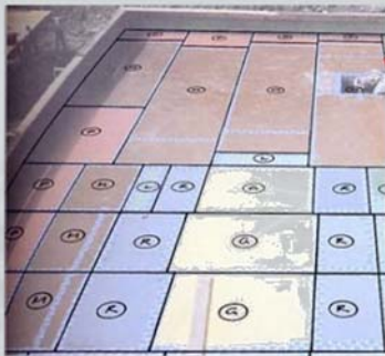
Laying of pads at building foundation according to load distribution
